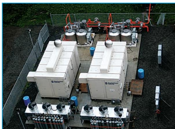
**figure 3.** The 26th Ward fuel cell installation with two 200-kW fuel cells and auxiliary equipment during construction.
