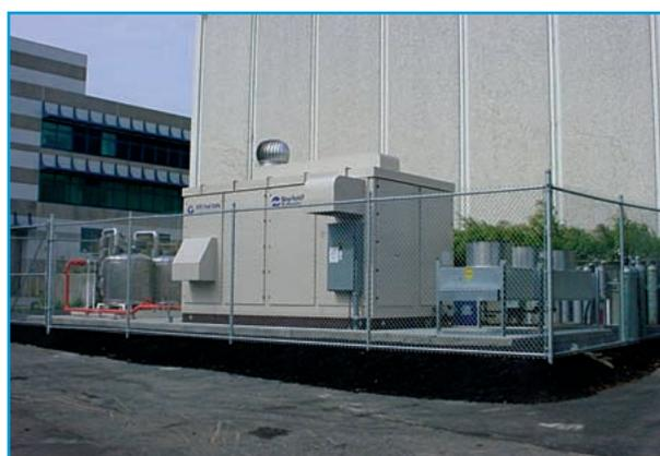
**figure 4.** Oakwood Beach fuel cell installation with one 200-kW fuel cell and auxiliary equipment.
