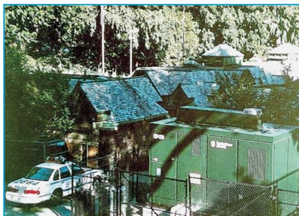
**figure 1.** The Central park fuel cell. It provided power during the August 2003 blackout.
